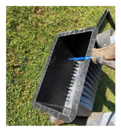
c. Core holes where required and position the bottom half into the hole. Do the same with the top half.
