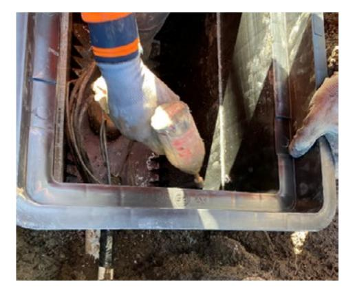
f. Screws shall be placed at maximum 100mm spacing
