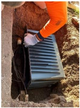
e. Place the top half Using the Telstra recommended self-drilling screws, start drill through horizontally and angle 45° down.
