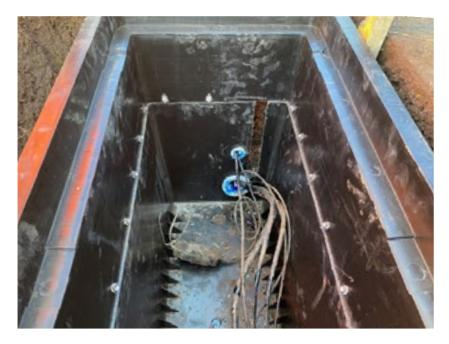
g. Use patch kits to seal the vertical cuts in the bottom section
