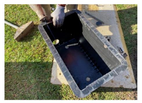
d. Place the bottom half of the pit around the cables
